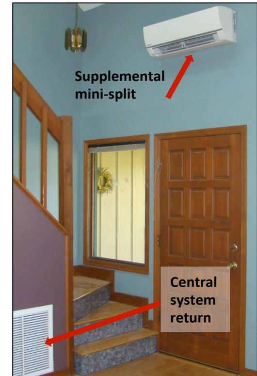
**Key Takeaway: Runtime of a low efficiency existing central system can be offset with a high efficiency supplemental system. Supplemental system provides redundancy if central system fails.**
